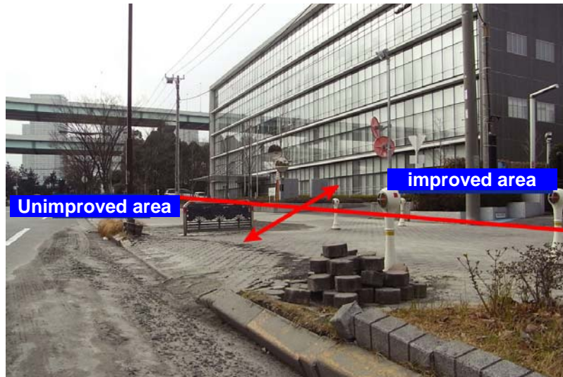
Photo 1: Successful ground improvement in Tatsumi area
