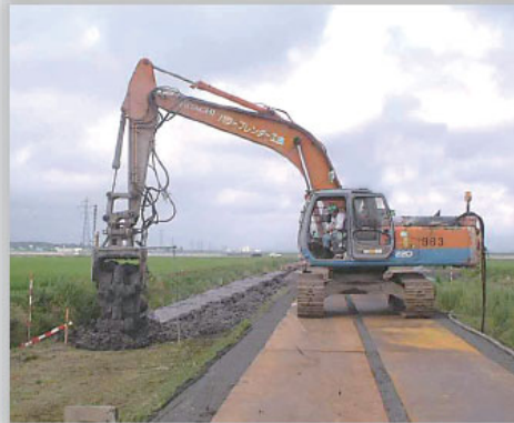
Stability increase for Road embankment
