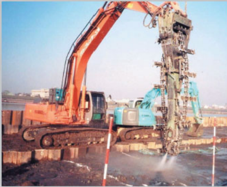
Liquefaction mitigation for River Dike
