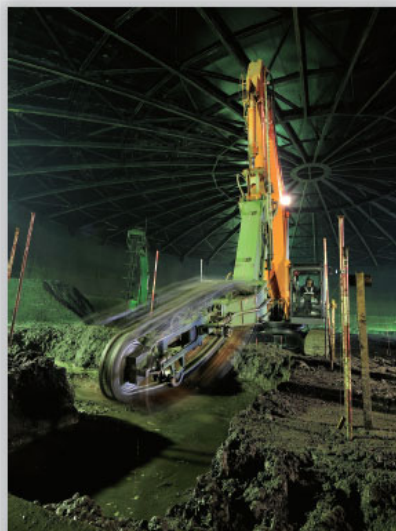
Overhead clearance Restricted area
