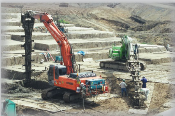
Stability Increase for high embankment
