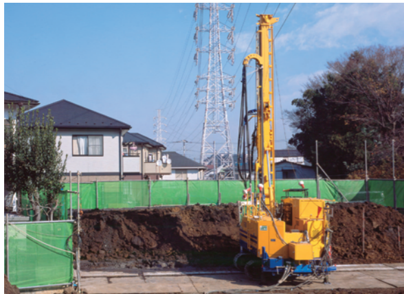
The use of compact construction equipment allows for construction work at locations with restrictions on the available space or height.
